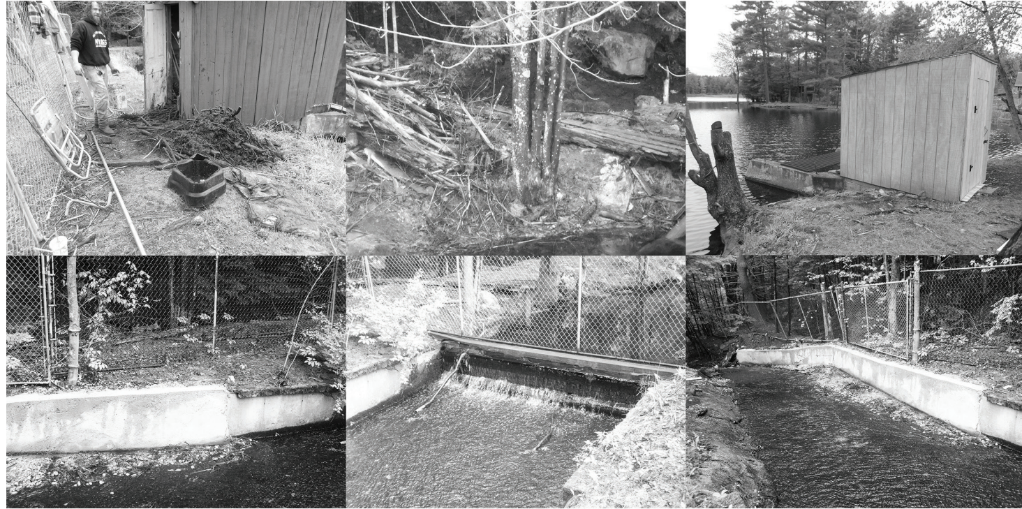
The Dam Project
